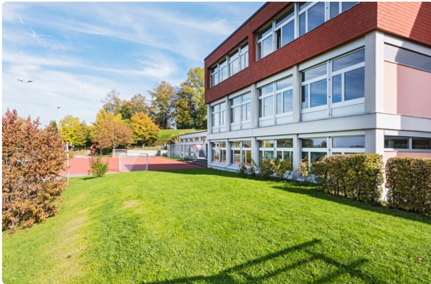
School building Allenwinden
