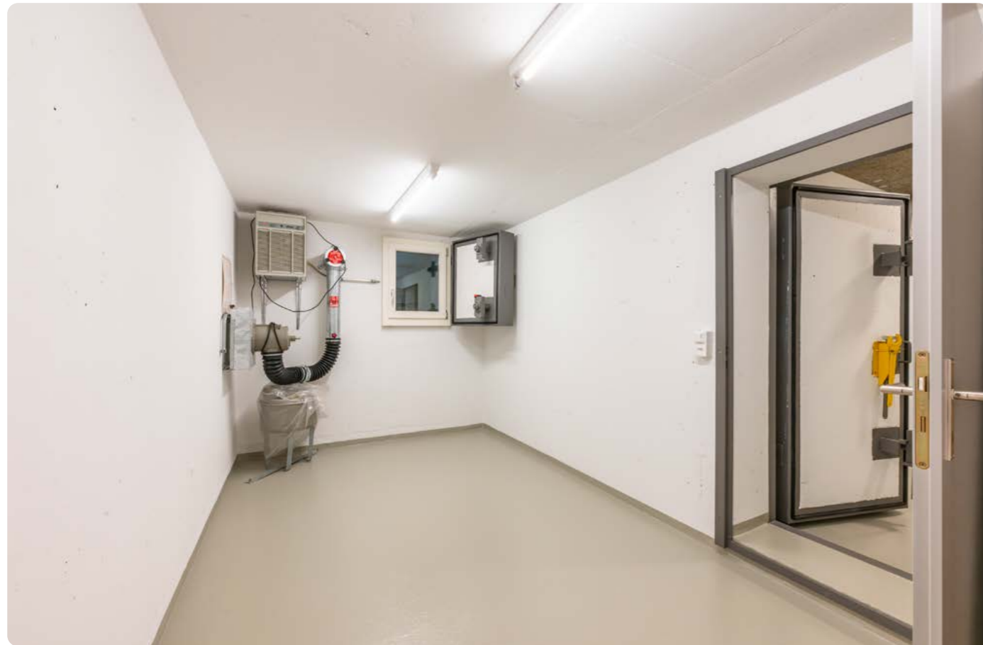
Cellar/Air-raid shelter on the basement level
