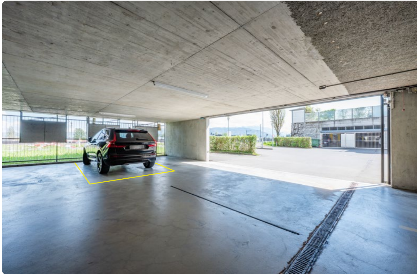
Underground garage parking space no. 2
