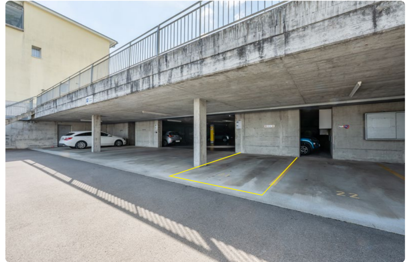
Covered external parking space (according to regulations no. 86) Marking no. 21
