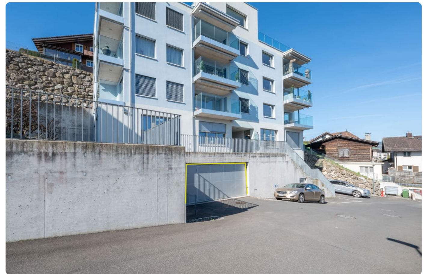
Entrance to the underground garage right next to the building
