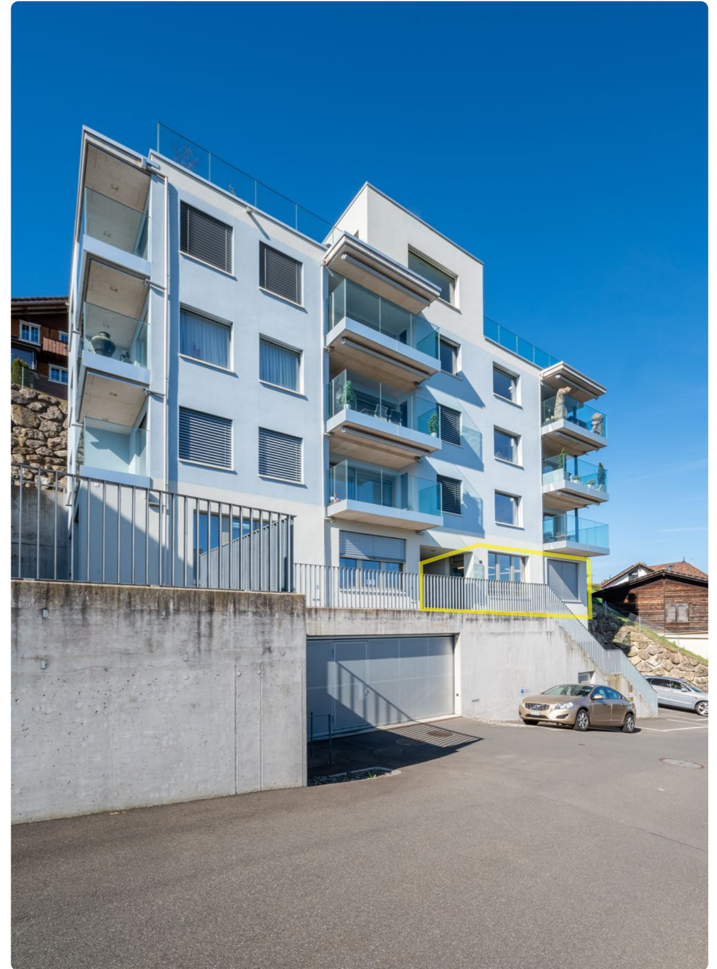
Building P96 West with the office on the ground floor
