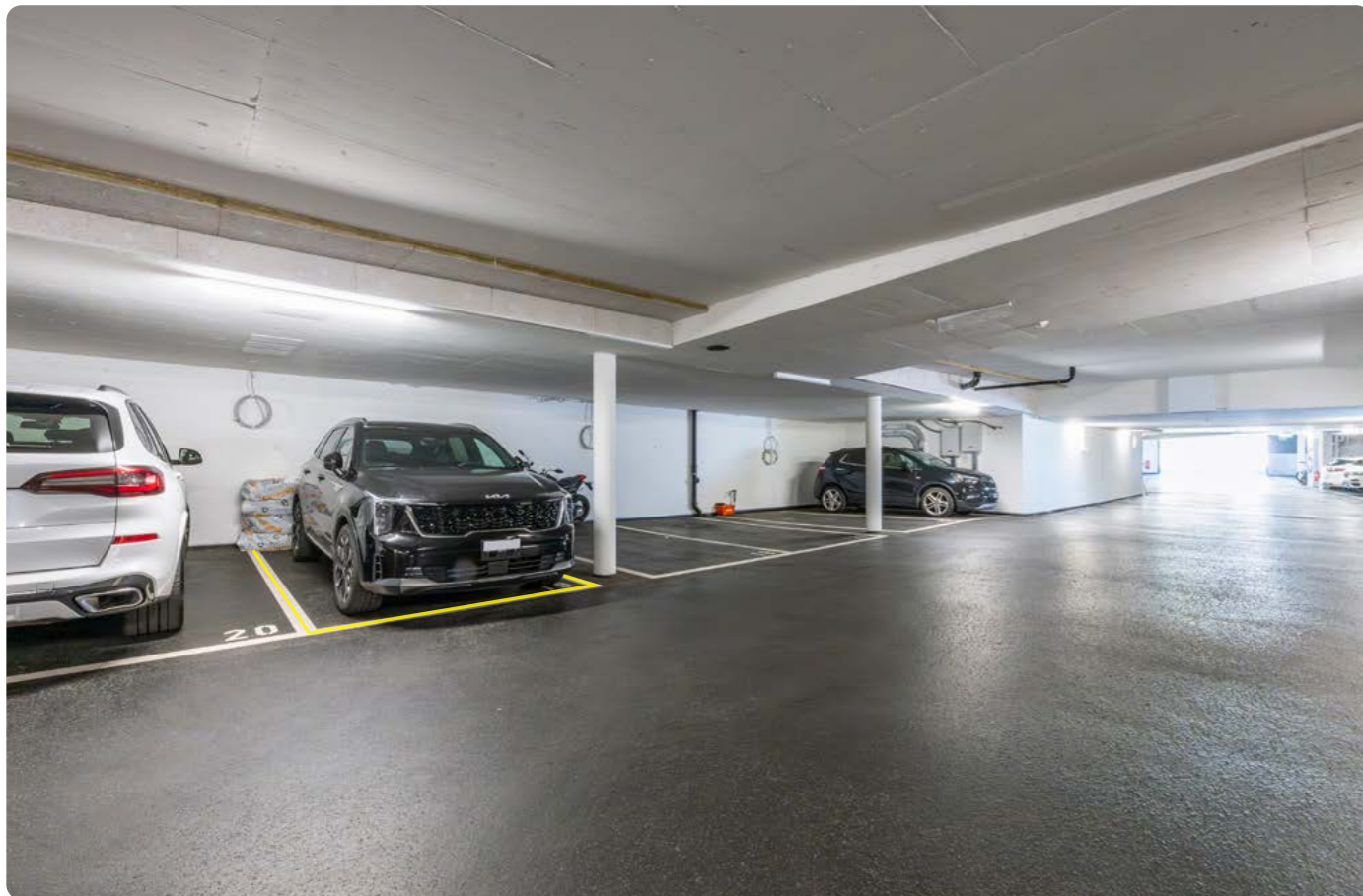
Underground garage parking space no. 19 with pre-installed e-car charging station
