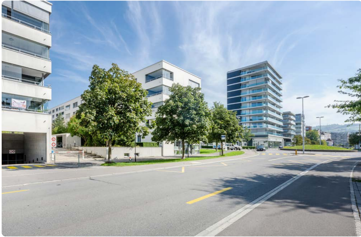
Access via Feldstrasse
