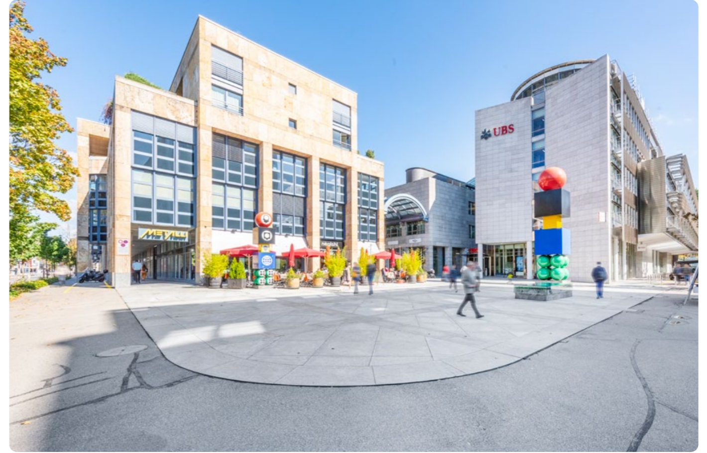
Metalli shopping centre Zug
