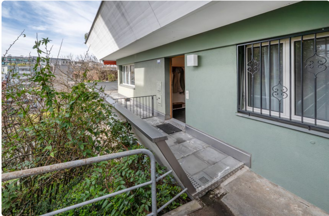
Entrance area of building 7h
